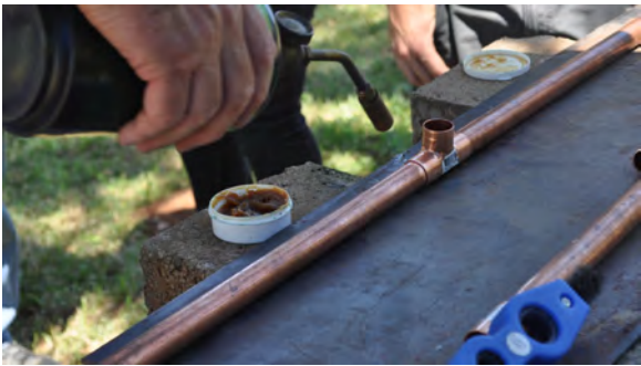
Soldering Copper Fittings
